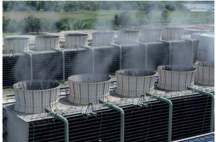
Typical open cooling towers
